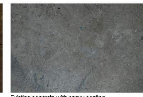
Existing concrete with epoxy coating
