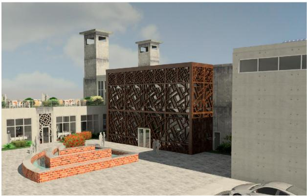
Shading of the south façade; the wooden entry in the façade with big and small patterns is inspired by "the *mashrabiya*," which is an old Arabic technique to cool interior spaces and to minimize the amount of light entering the building. The small pattern in the top of the walls is used to ventilate the space, and it has sensors to close the glass windows behind the wooden patterns automatically.
